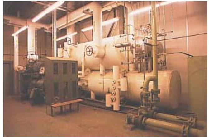
The latest computerized central ammonia refrigeration technology installed in the freezer addition is more costeffective, significantly reducing energy consumption.
